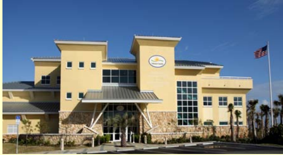
Beach Administration Headquarters
