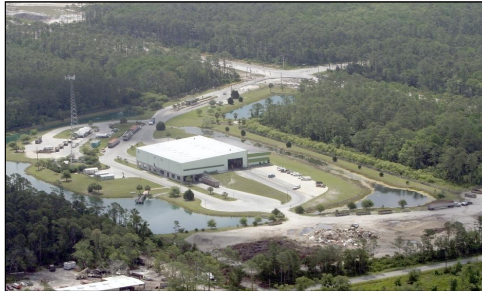
West Volusia Transfer Station
