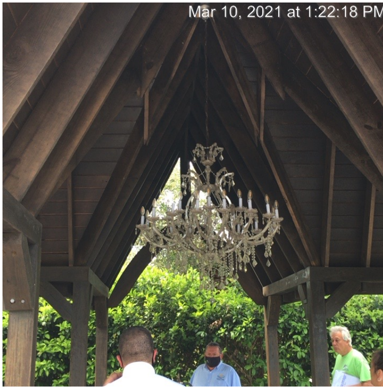
Close up of Unpermitted Accessory Building
