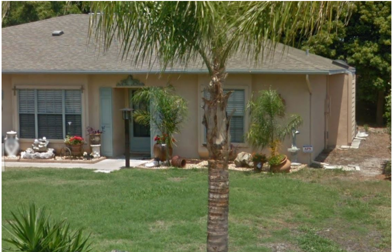
View of east façade off-set.
