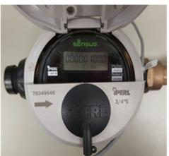
Compare the first four numbers to the read on your bill. Current meter reading \_\_\_\_\_\_ - meter reading on bill \_\_\_\_\_\_ = \_\_\_\_ gallons used since your bill date. If the leak indicator is indicating water usage, locate your house valve and turn it off. If the meter stops spinning, the leak is in
