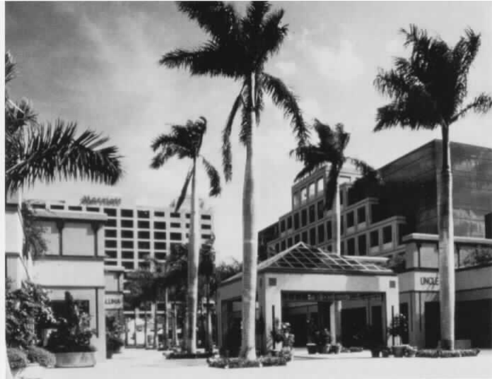
The three uses—retail, office, and hotel—located on this 28-acre suburban site are integrated by a pedestrian promenade and a landscaped courtyard.
