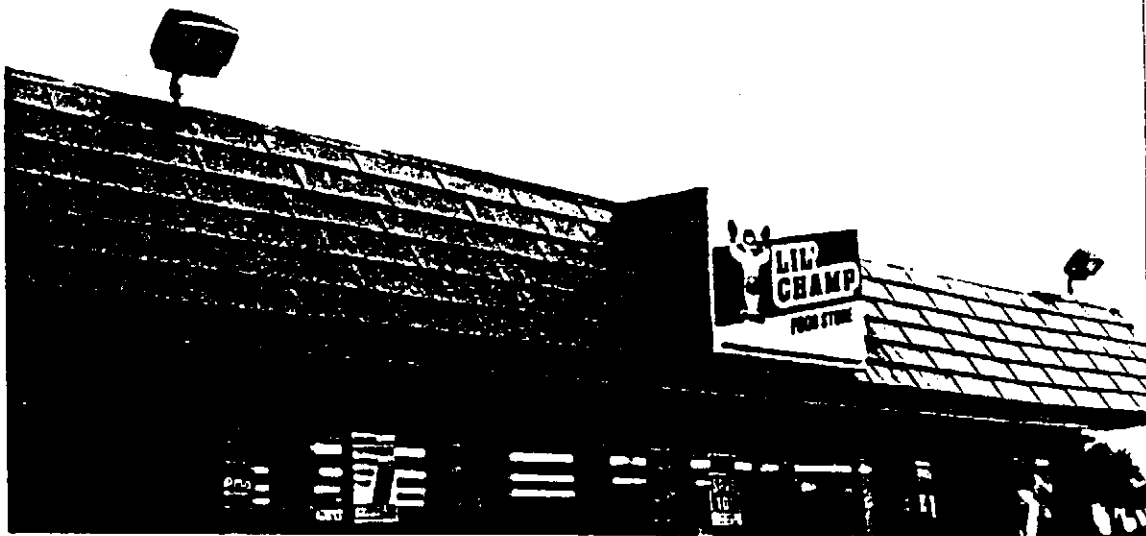
Figure 6 Unshielded Roof Mounted Security Lights
