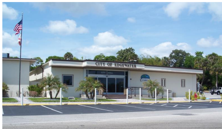
Photo: Edgewater's City Hall Building is partially located within the 100-Year Floodplain
