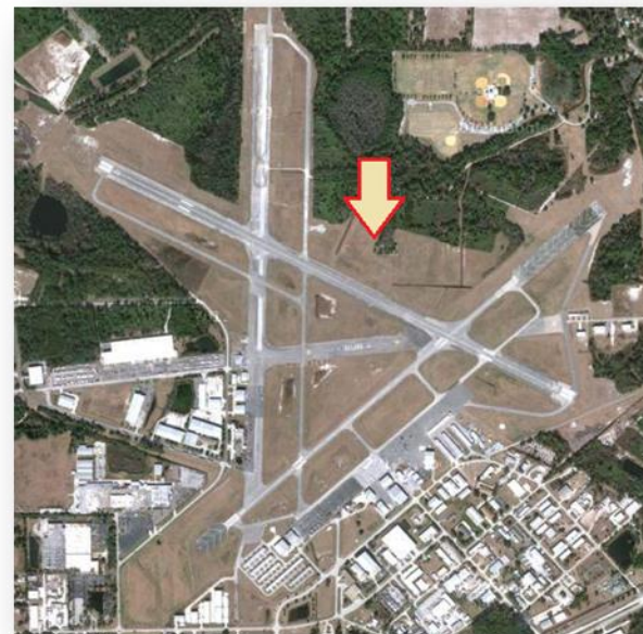
Photo: DeLand Municipal Airport is located within the 100-Year Floodplain in Volusia County
