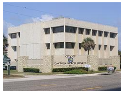
Photo: The Daytona Beach Shores City Hall building is at risk for storm-surge damage
