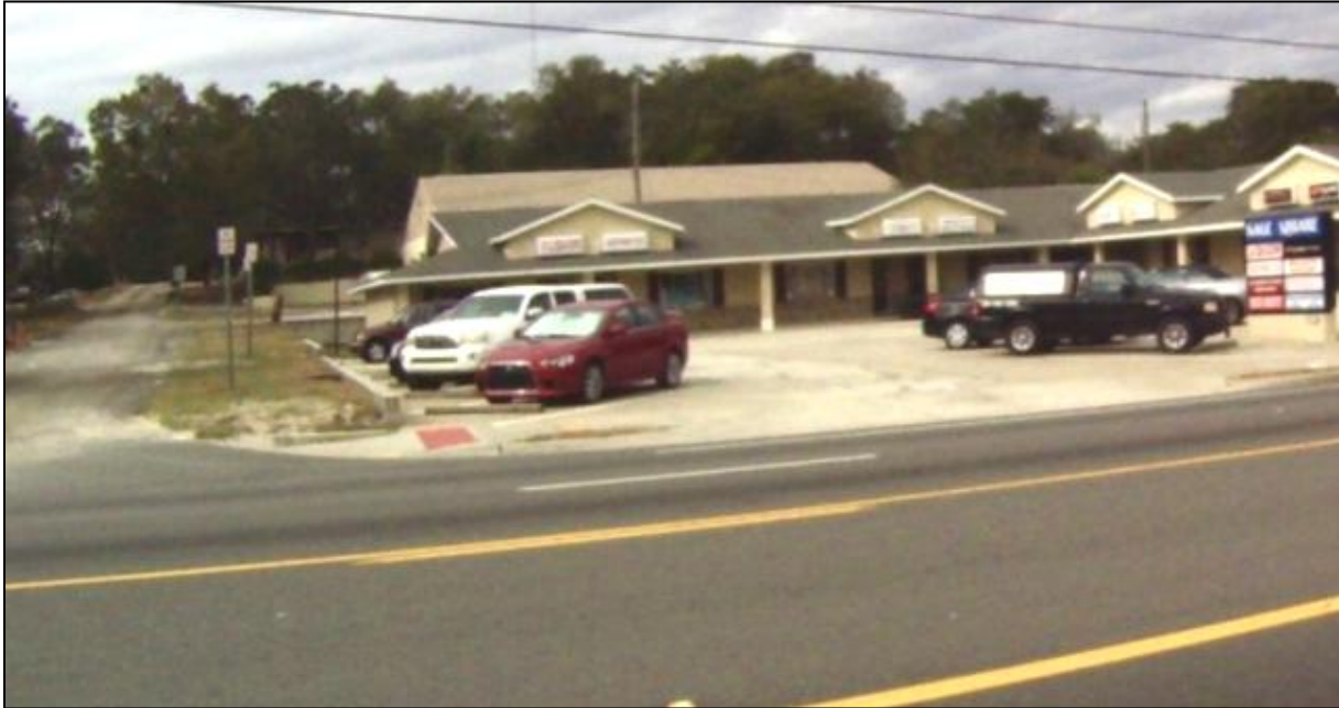
US 17-92 (Volusia Ave.) - No streetscaping, narrow sidewalks, no bicycle lanes, typical drainage swales
