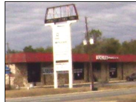
US 17-92 (Volusia Ave.) - Deteriorating site
