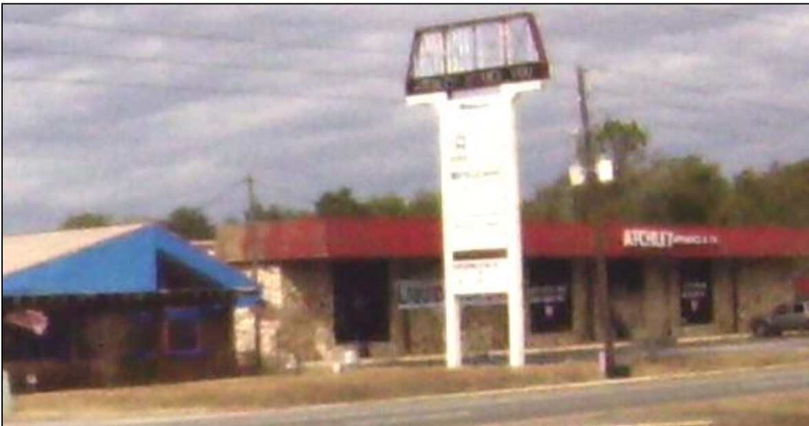
US 17-92 (Volusia Ave.) - Poor site maintenance
