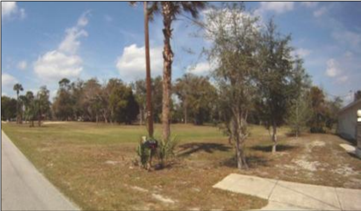
E. Blue Springs Ave. – Discontinued sidewalk , limited streetlights
