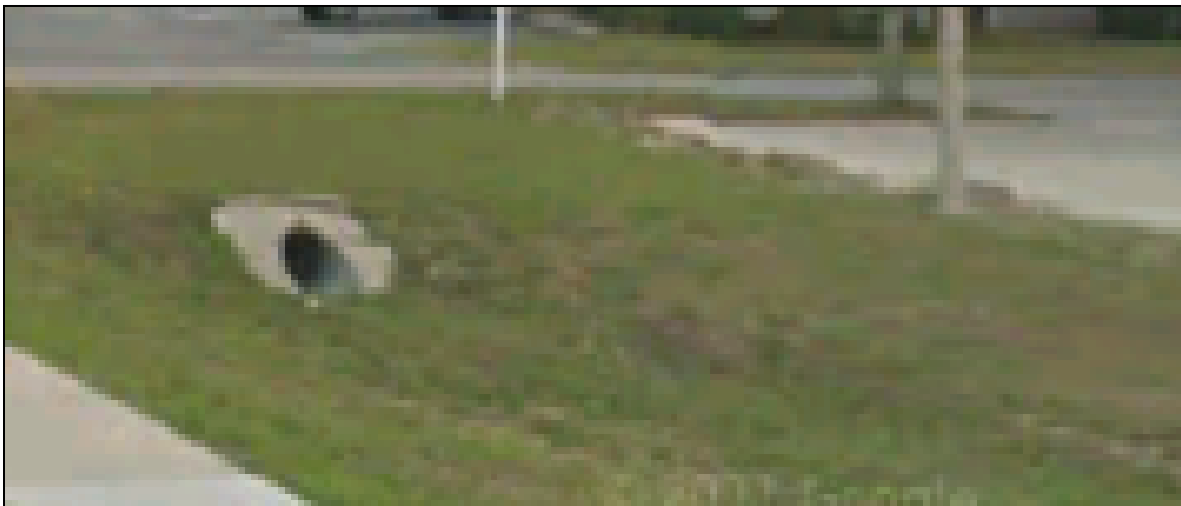
US 17-92 (Volusia Ave.) - Stormwater culverts and drainage basins
