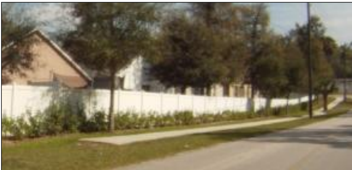
E. Ohio Ave. - Discontinued sidewalk, limited pedestrian lights
