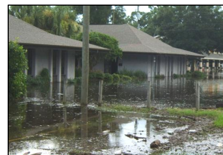
E. Elm Ave. at US 17-92 (Volusia Ave.) - Deteriorating infrastructure
