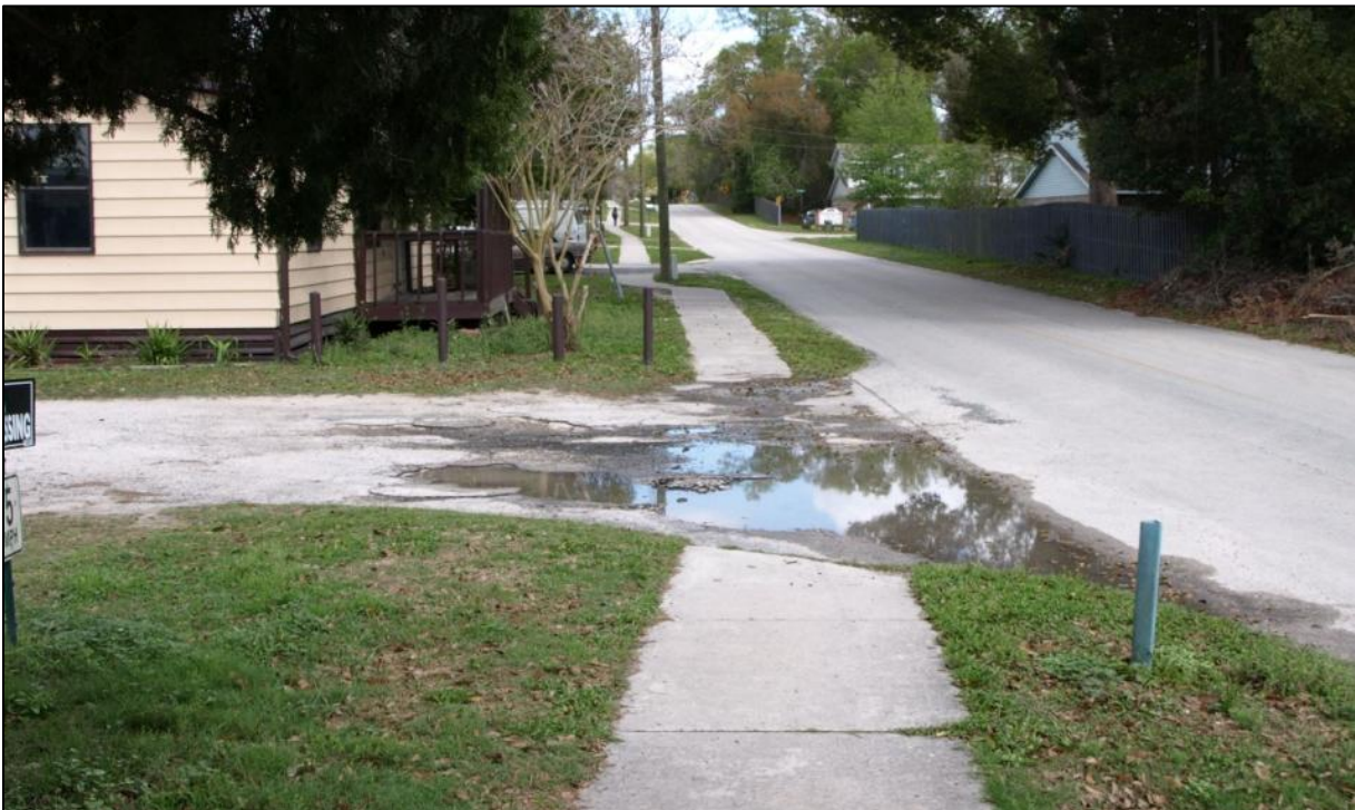
E. Ohio Ave. - Standing water
