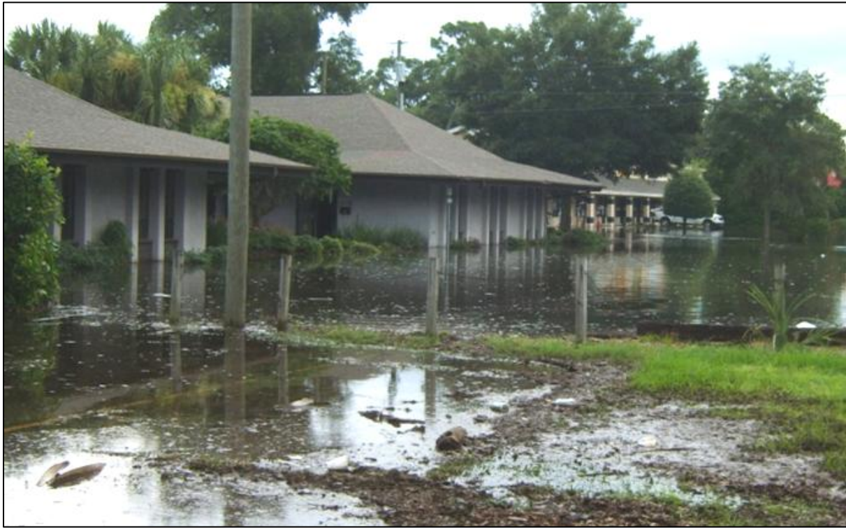
E. Elm Ave. at US 17-92 (Volusia Ave.) - Flooded businesses (Photos provided by City)
