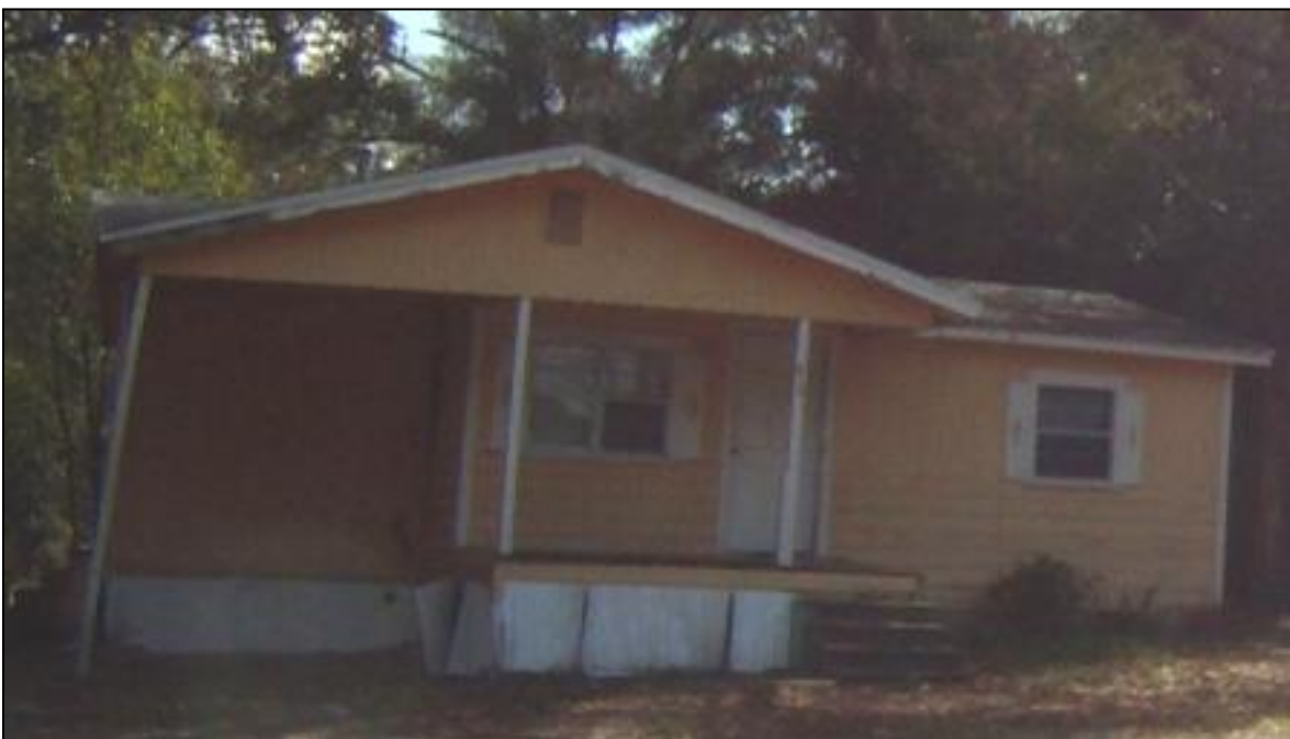
S. Orange Ave. - Home not well maintained
