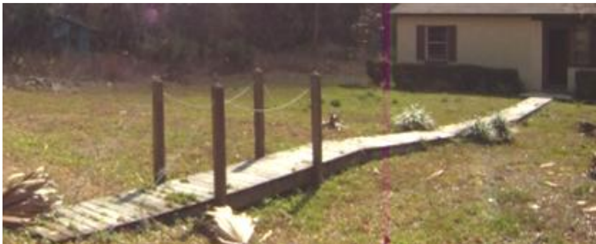
Banana Ave. - Drainage swale
