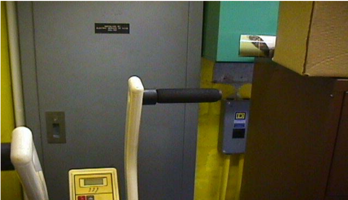
Blocked electrical panel.
