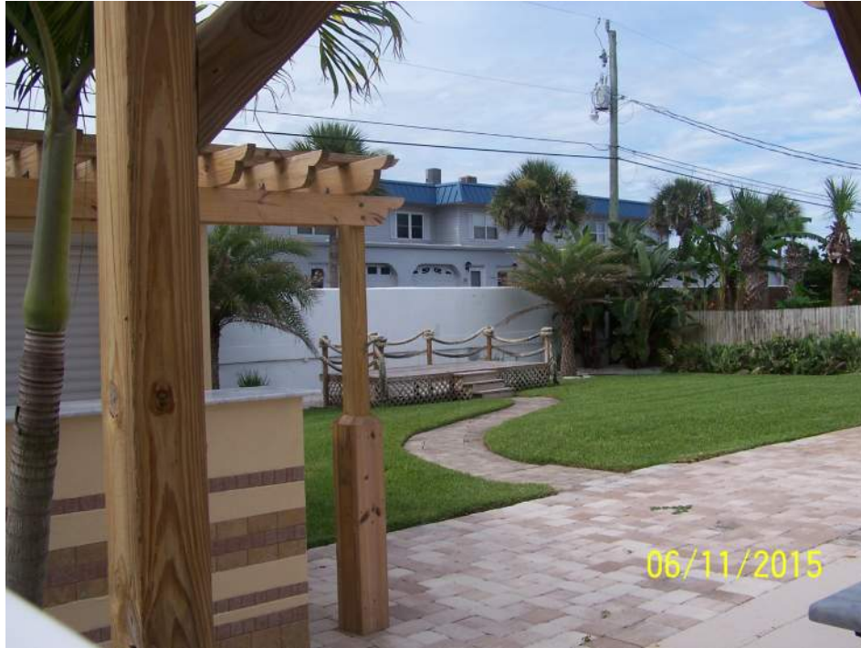
Wooden deck at the rear property line. The deck has been cut so that it no longer rests directly up against the fence line.
