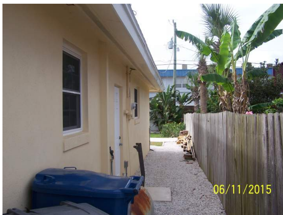
Western property line, depicting the 5.8-foot setback for variance 2. The plastic shed shown on the survey has been removed.
