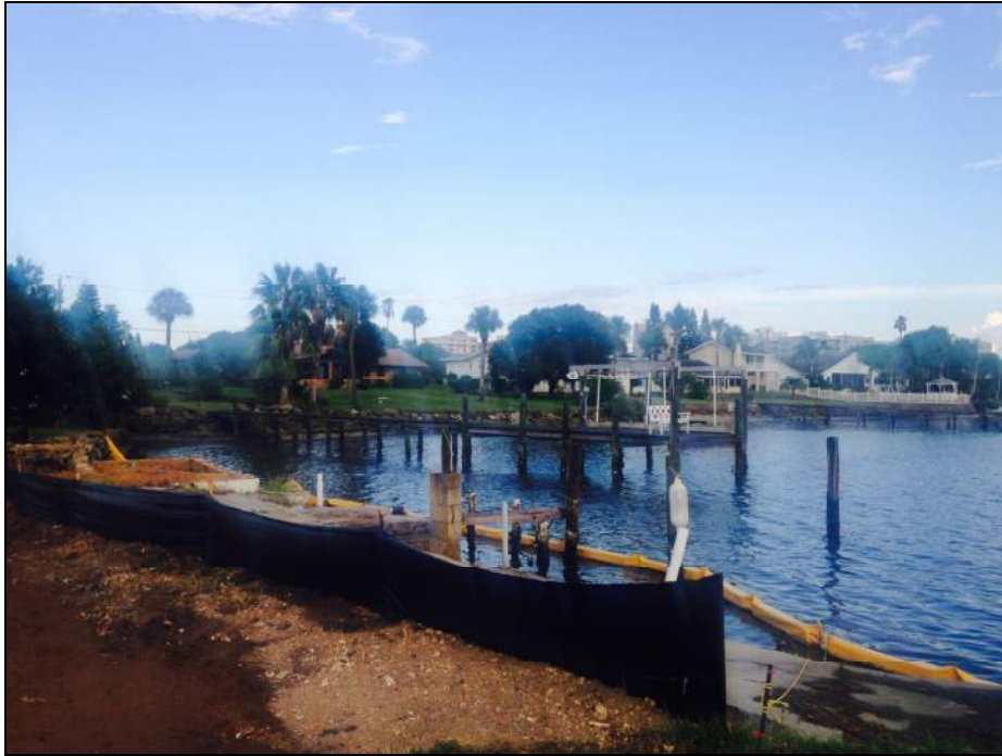
View of the southern shoreline from the construction area.
