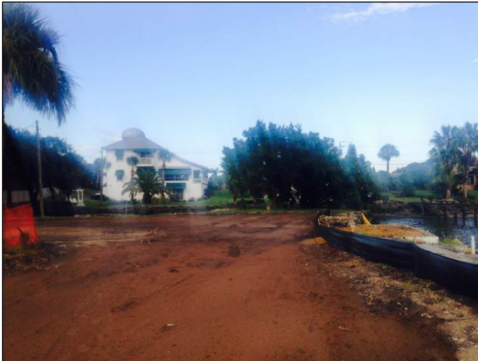
View of the eastern shore from the construction area.
