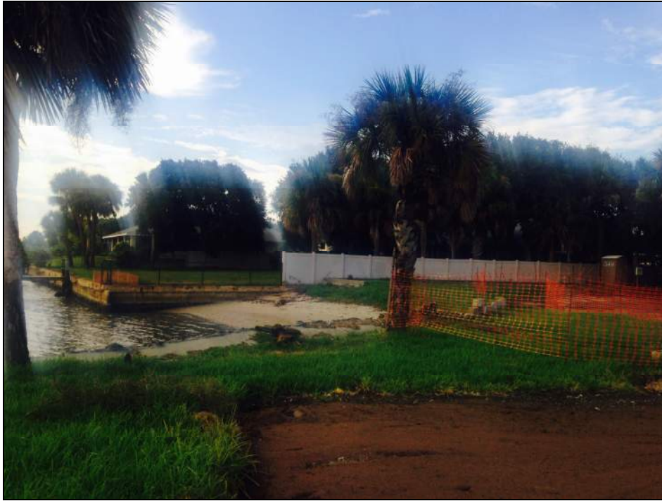
View of 2806 S. Peninsula Drive (property to the north) from the construction area.
