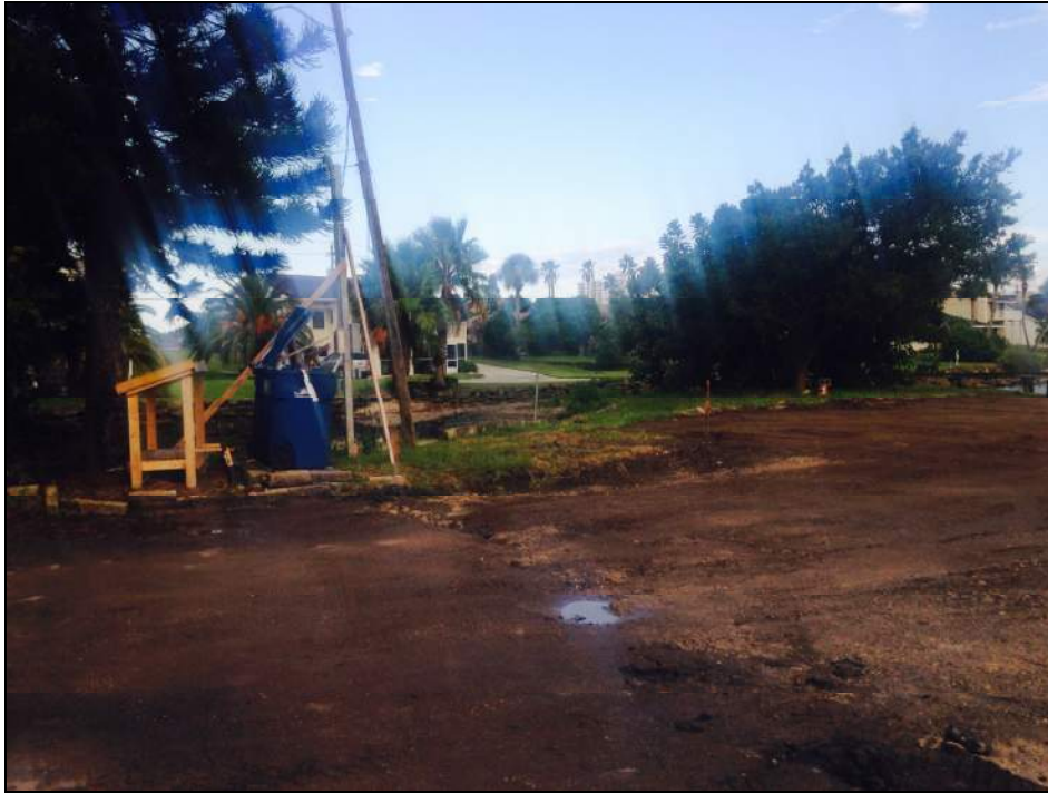
View of 2814 S. Peninsula Drive, from the construction area.
