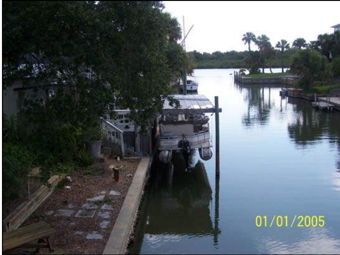
Photo of boat house extending into canal, of property on other side of east neighbor. Structure is on the common property line.
