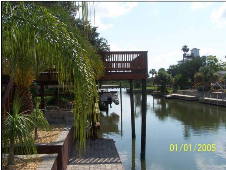
Photo taken from seawall, showing 6-foot deck extension into canal.
