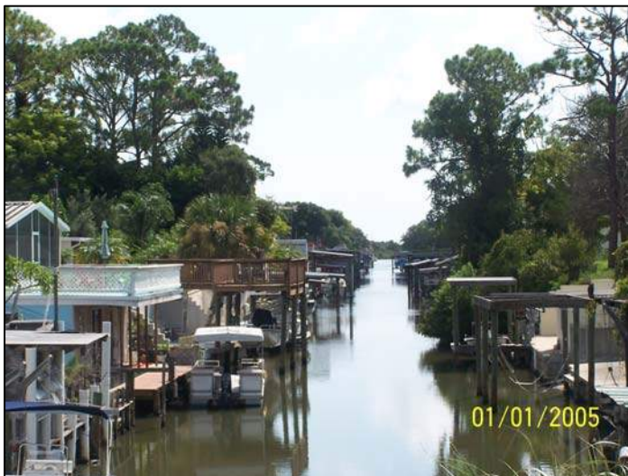
Photo taken at west end of canal, looking east. Shows the number of structures extending into the water. Very few of them appear to meet the 15-foot side setback requirement.
