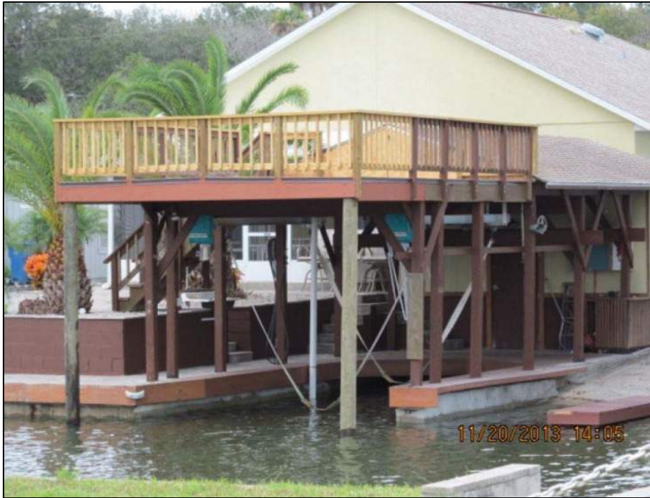
Photo taken by Code Enforcement in 2013, from across the canal.
