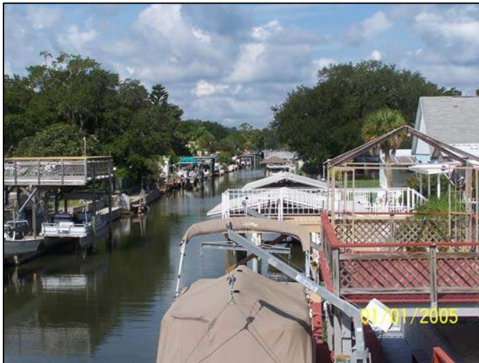
Photo of canal, looking west from subject property's deck. Shows the number of structures extending into the water. Very few of them appear to meet the 15-foot side setback requirement.
