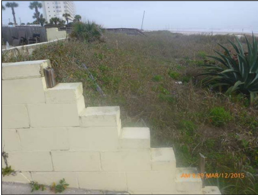
Masonry retaining wall (seawall) with dune vegetation. You can see the stormwater water pipe (white area) near the agave plant.
