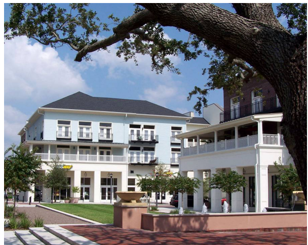
Baldwin Park, a traditional town development in Orlando, integrates retail, commercial, and a variety of residential uses with public spaces. To ensure a high level of walkability, the roadways form an interconnected network and most daily needs are located within easy walking and biking distance. One-half of the site (450 acres) is conserved open space.
