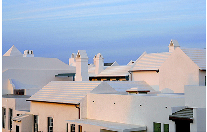
Alys Beach, a mixed-use community in Walton County, utilizes a full range of building practices, including positioning most homes to allow passive heating from the sun and cooling from the Gulf breezes. Sun-reflecting white exterior walls and roofs and masonry construction add to the community's energy-efficiency.
