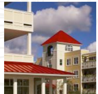
The Prairie Crossing Charter School building has attained Energy Star's highest rating for energy efficiency
