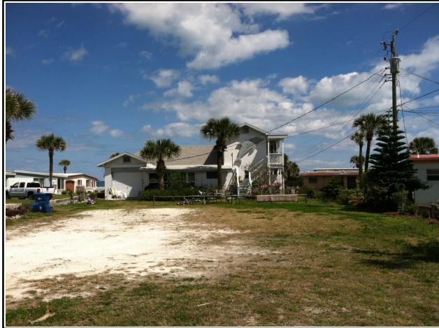
Front View of Dwelling Looking East
