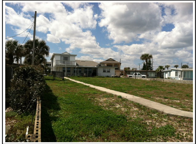
Rear View of Dwelling Looking West
