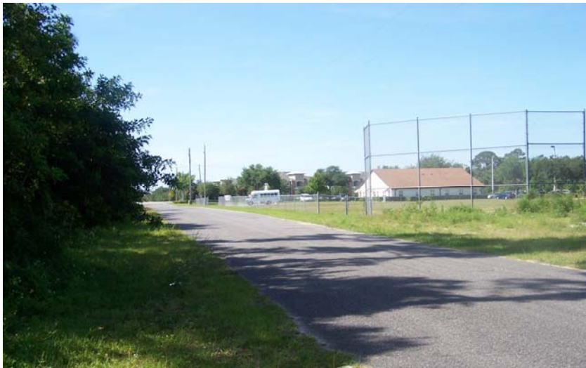
View of Old Kings Road, looking south from the subject property.
