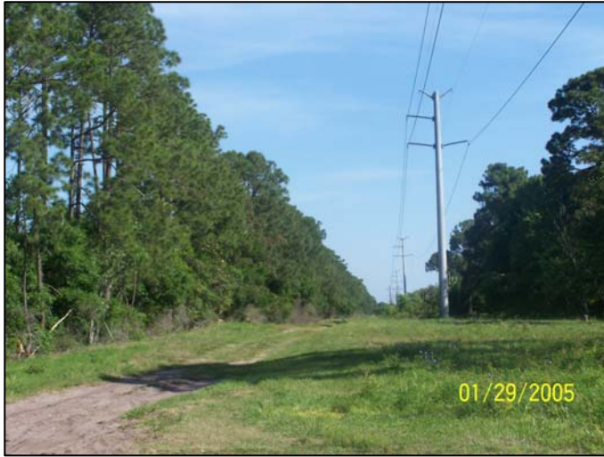
View of trees bordering drainage ditch and 100-foot FPL easement between subdivisions.
