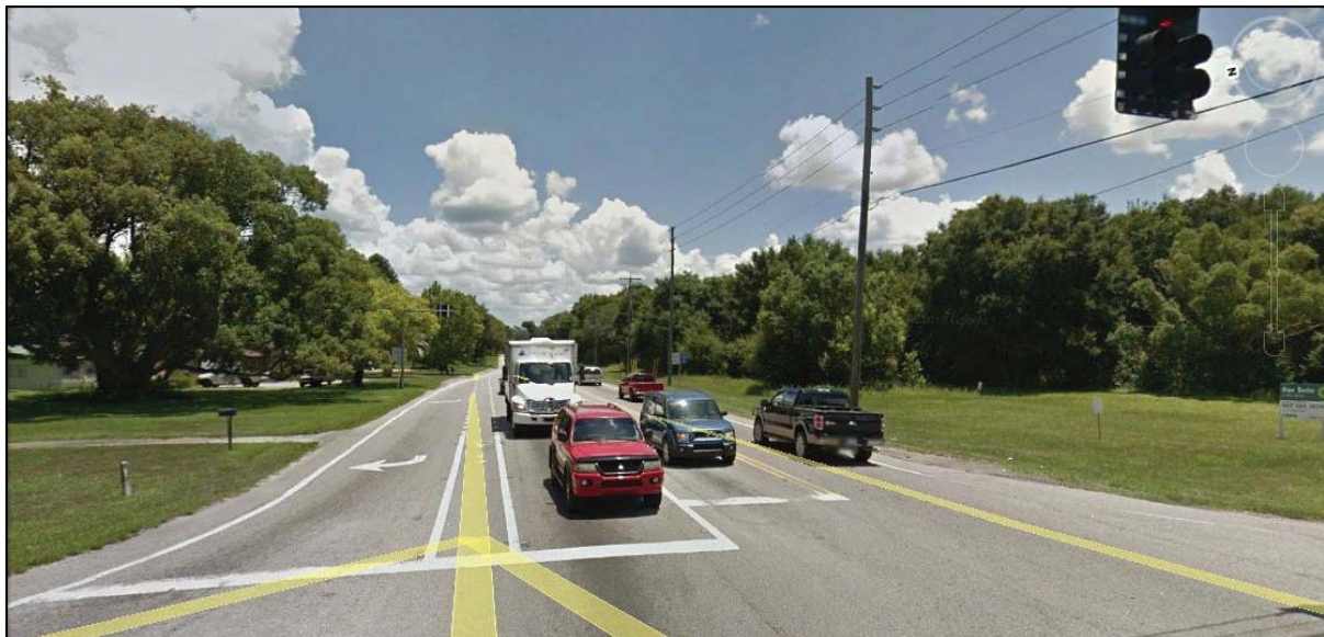
SR 44/Kepler Rd. intersection, looking east
