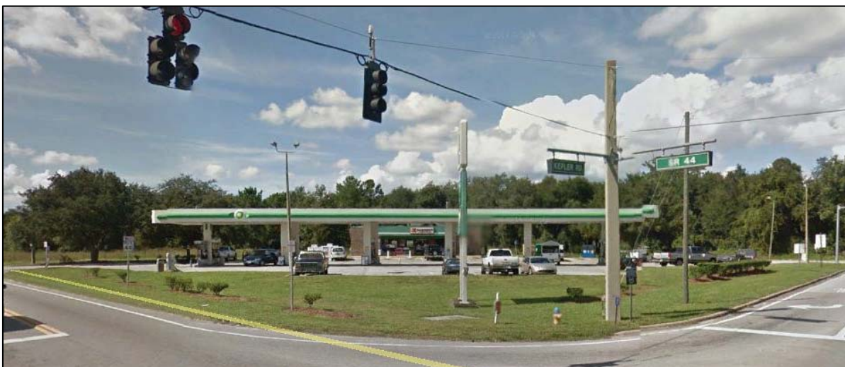
Existing BP/Kangaroo convenience store, NW corner of SR 44/Kepler Rd.
