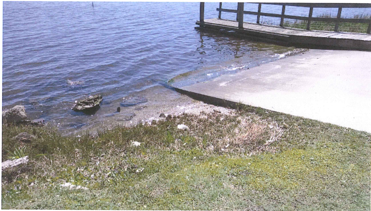
Existing boat ramp
