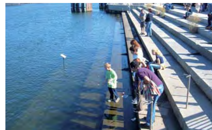
BELOW: Steps to the river along the promenade allow people to directly interact with the water.
