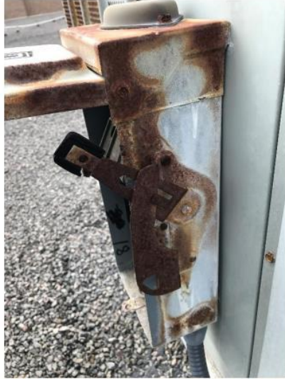
Photo 21: Deteriorating disconnecting means for HVAC equipment. (typical)
