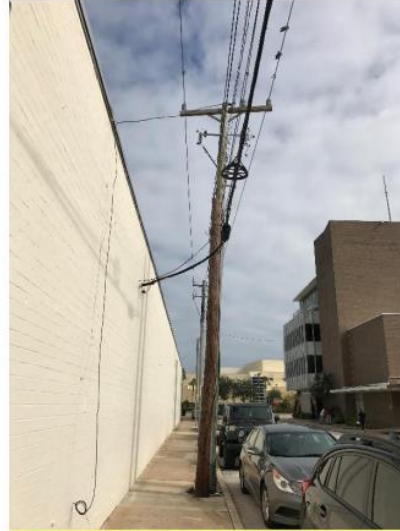
Photo 18: Existing overhead electric serving fire pump.
