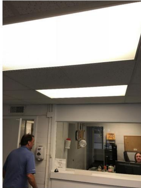
Photo 14: Typical 2x4 prismatic troffer throughout office building.
