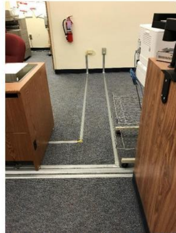
Photo 2: Communication and power wiring on floor.
