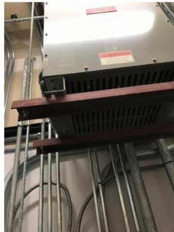
Photo 16: Typical hung mounted transformer.
