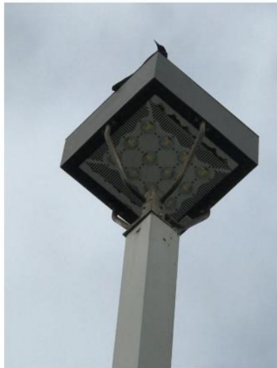
Photo 24: LED site lighting fixture.
