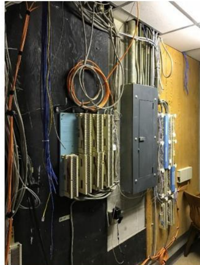
Photo 17: Typical communications backboard.
