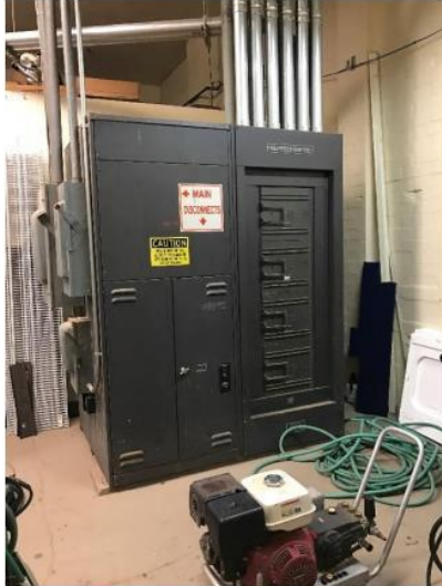
Photo 5: Existing 2000 amp switchboard.
