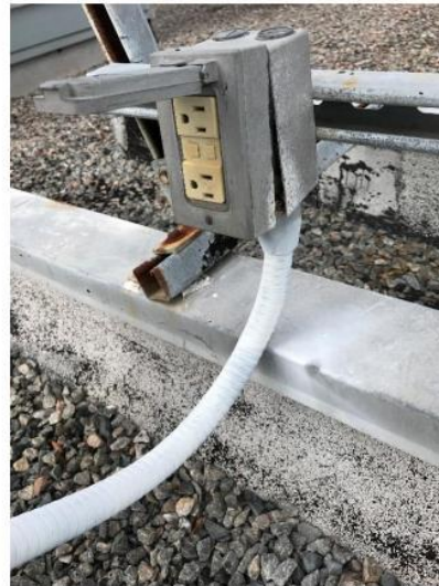
Photo 24: Separated wiring device.
