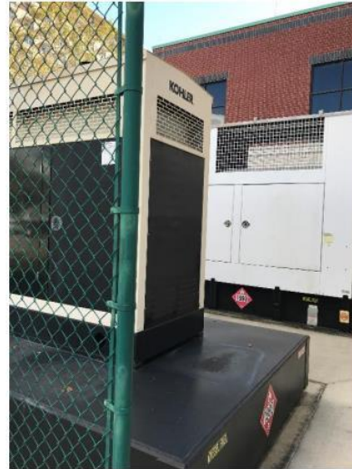
Photo 2: Existing standby generators.
