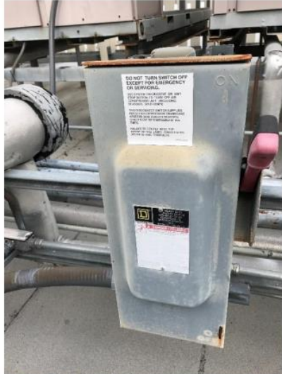
Photo 182: Existing disconnecting means for mechanical equipment.
