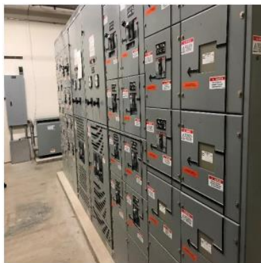
Photo 3: Existing 3000 amp switchboard MDP-A and MDP-B.
