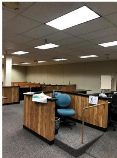
Photo 8: Existing courtroom lighting prismatic troffer.
