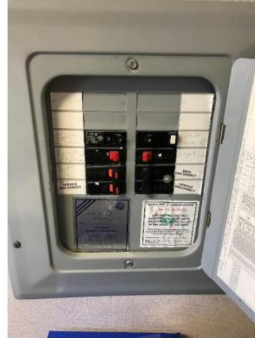
Photo 9: Existing main service panel for Public Defender trailers.
