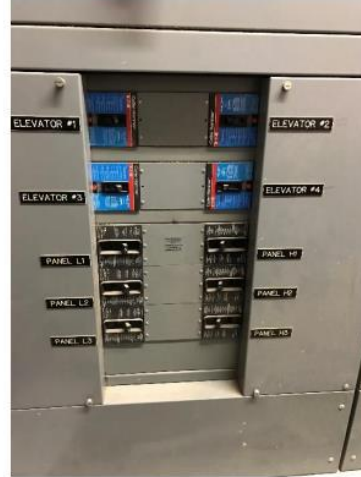
Photo 2: Existing distribution section in MSB.
