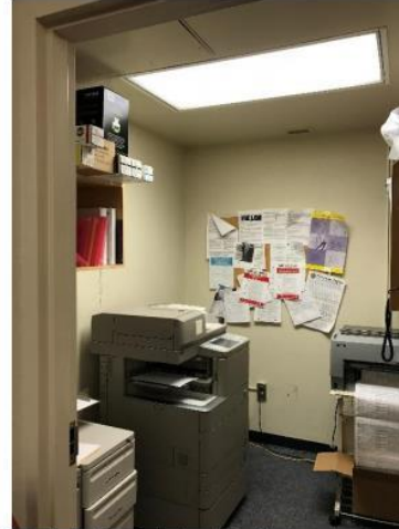
Photo 6: Existing 2x4 prismatic troffer throughout spaces.
