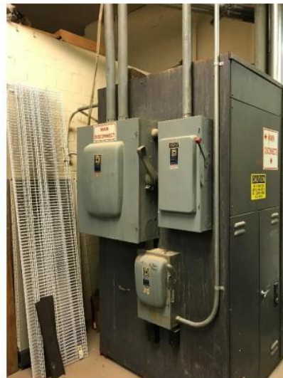
Photo 4: Existing 2000 amp switchboard with disconnect tapped off the switchboard buss.
