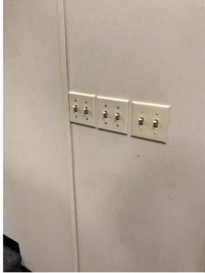
Photo 9: Existing manual lighting controls.
