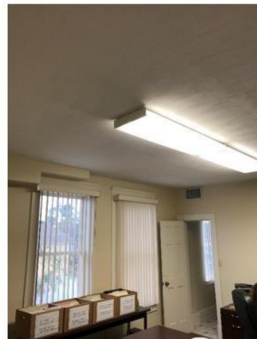
Photo 12: Existing 4 ft. wrap around light fixture.
