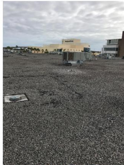
Photo 20: Roof with no lightning protection.
