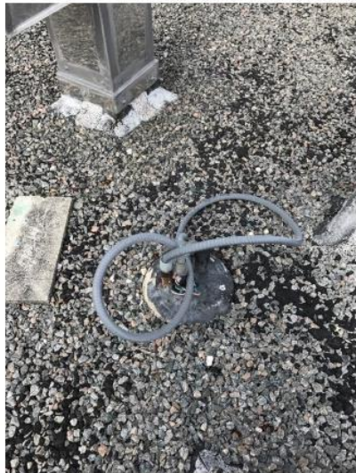
Photo 23: Separated fitting and conductors.
