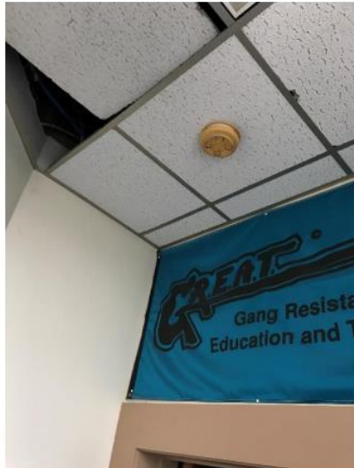
Photo 3: Existing smoke detector.
