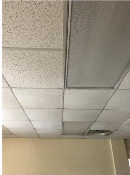
Photo 6: Existing 2x4 prismatic troffer throughout building. typical)
