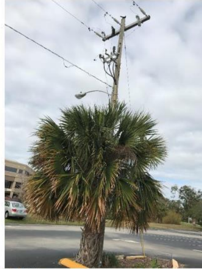
Photo 2: Existing overhead primary serving Admin Building.
