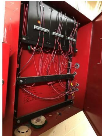
Photo 12: Existing fire alarm terminal cabinet.
