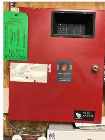
Photo 8: Existing fire alarm control panel.
