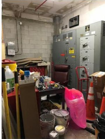
Photo 1: Existing 1600 amp, 277/480V, 3 phase, 4 wire main switchboard in main electrical room.
