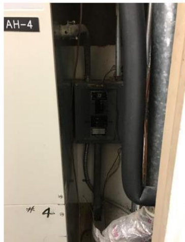
Photo 11: Existing disconnect means with clearance issues.
