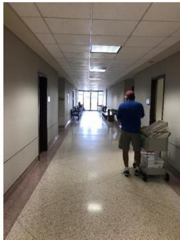
Existing 2x2 parabolic light fixtures.
