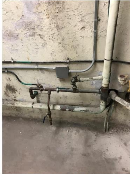
Photo 10: Existing grounding.
