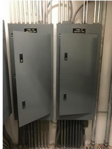
14: 120/208V panels in floor electrical rooms.
