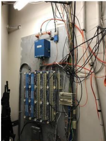
Photo 7: Existing punch down.
