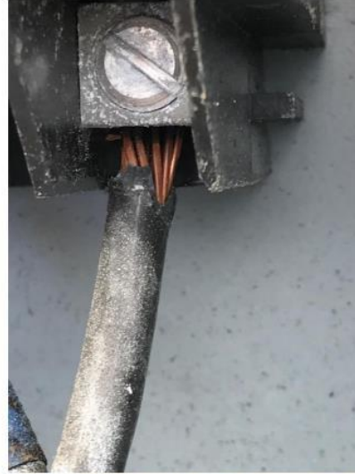
Photo 22: Loose termination on HVAC disconnecting means.
