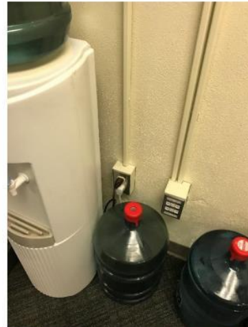
Photo 8: Surface mounted devices. (typical)
