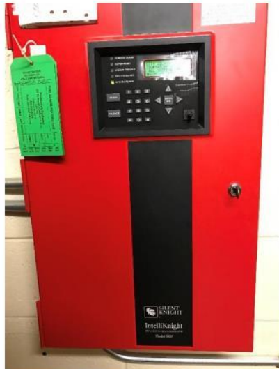
Photo 11: Existing Fire alarm Panel.
