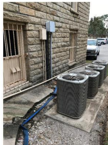
Photo 4: Missing 120V GFI receptacle require per code.
