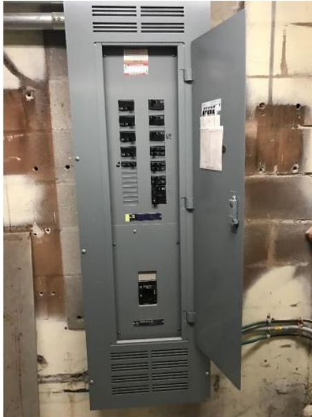
Photo 9: Existing main distribution panel located in basement.
