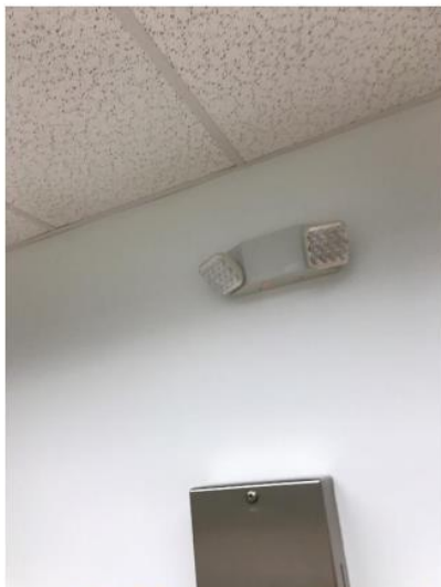
Photo 7: Existing emergency lighting. (typical)
