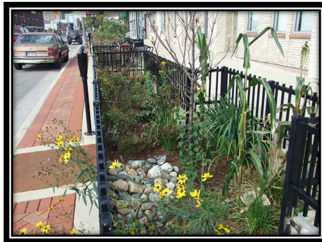
Figure 75: Planter boxes capture and treat much of the stormwater from roads and sidewalks.
