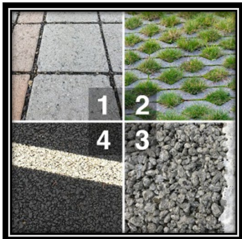
Figure 32: 1 – Permeable Pavers, 2 – Grass Pavers, 3 – Pervious Concrete, and 4 – Porous Asphalt
