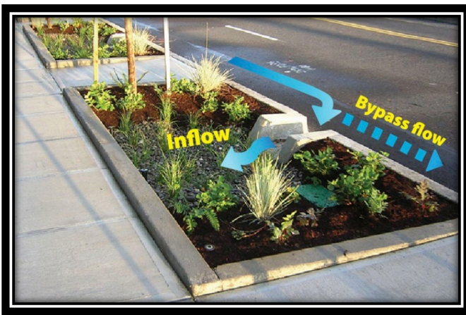
Figure 27: Curb cut facilitates the entry of street runoff. If it reaches capacity, excess water will be directed to a bypass the system.
