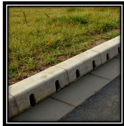
Figure 30: Perforated Pre-Cast Curbs
