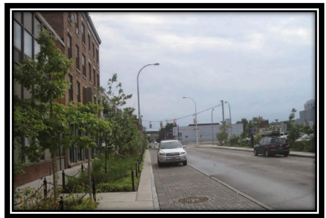
Figure 28: A permeable interlocking concrete paver parking lane is adjacent to a sidewalk planter.
