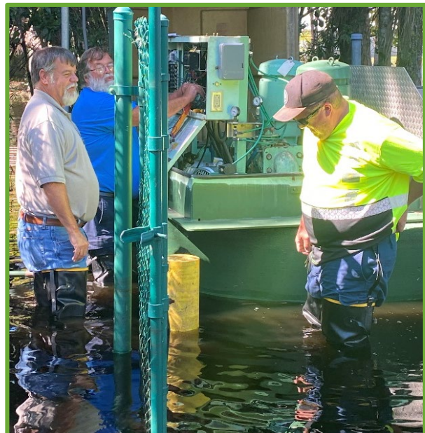
Field operations staff working to restore wastewater lift station service in a flooded area following a hurricane.
