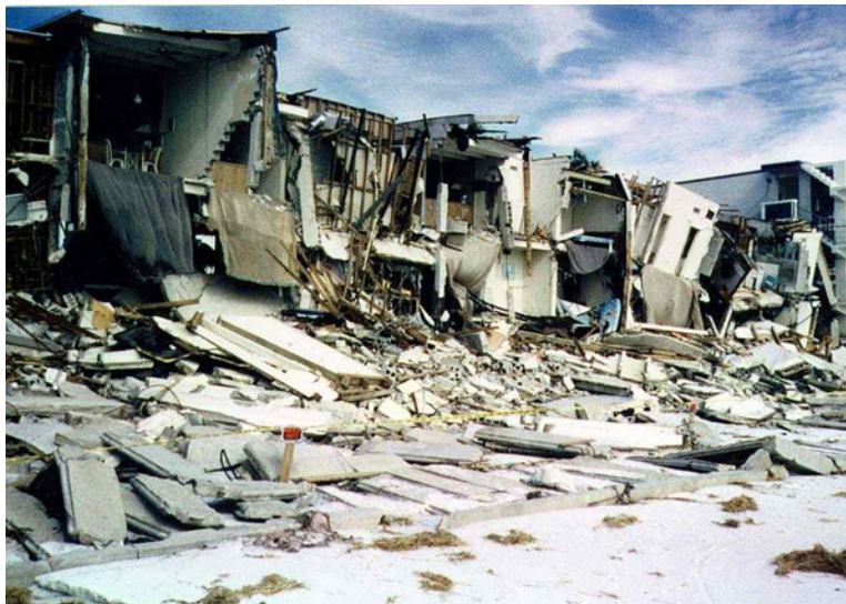
Figure 4.18 Storm Damage at Panama City Beach Caused by Hurricane Opal (Leadon et al., 1998)
